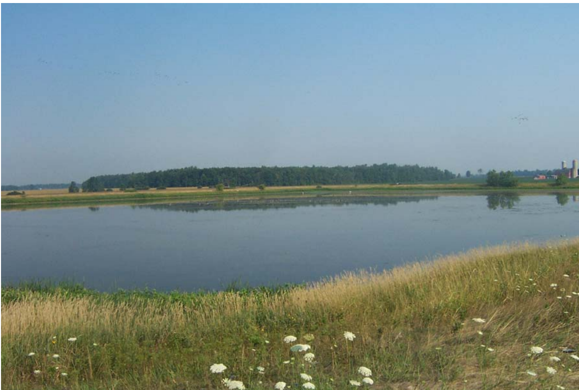
This photo displays one of the four Aylmer Sewage Lagoon Cells.
