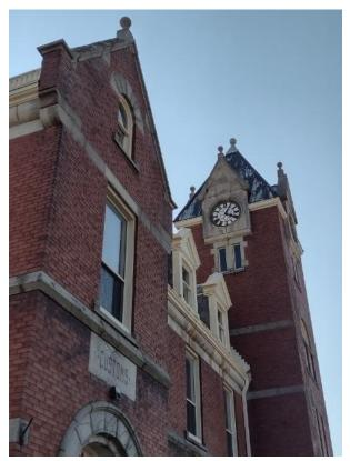
The Clock Tower requires upgrades to the roof and the brick work needs to be patched, repointed, and upgraded so that it does not become a safety hazard. As mentioned above, challenges to accessing and working in this area make it worthwhile to combine multiple projects in the general vicinity. Staff intend to provide Council with pricing options in late 2024 to early 2025 to commence structural works in spring of 2026 pending budget considerations.
