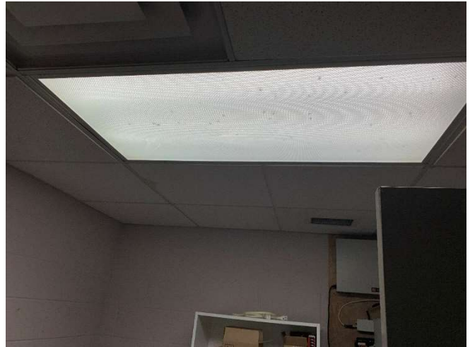
Water staining and possible damages were observed at the light fixture in the breath test room.
