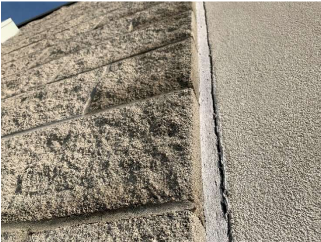
View of the failed sealant observed at an exterior wall transition located along the south elevation.
