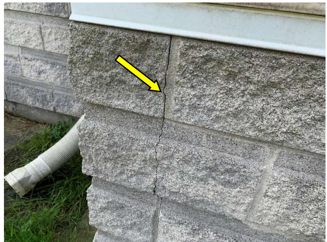
Minor cracking was observed in the split faced concrete block along the north elevation.
