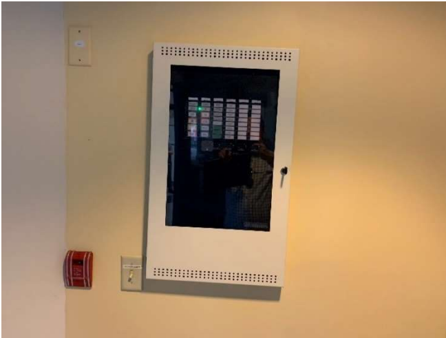
View of the fire alarm panel manufactured by Mircom.
