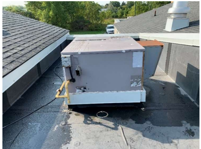
View of the package HVAC system located on the low sloped roofing at the north end of the building.
