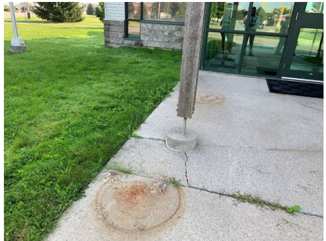
Settlement observed in the concrete pad surrounding the concrete pier at the main entrance.
