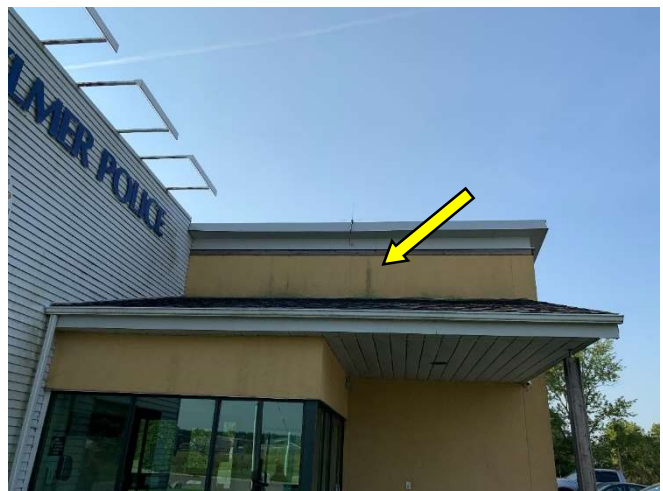
Severe staining was observed on the EIFS above the roof overhang at the main entrance.
