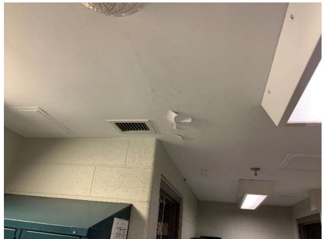
Damaged ceiling finishes observed above the holding cell area.
