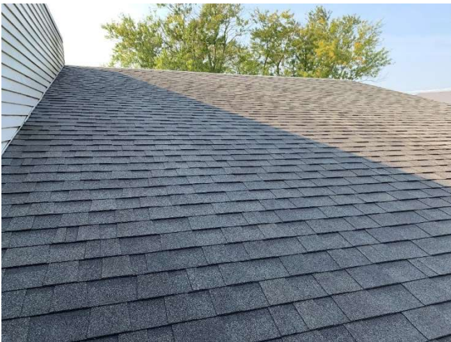
View of the asphalt shingle roofing observed at the south-west corner of the building.
