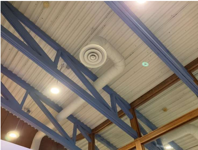
View of the pre-engineered wood truss roof framing at the corrugated steel decking observed in the meeting room.
