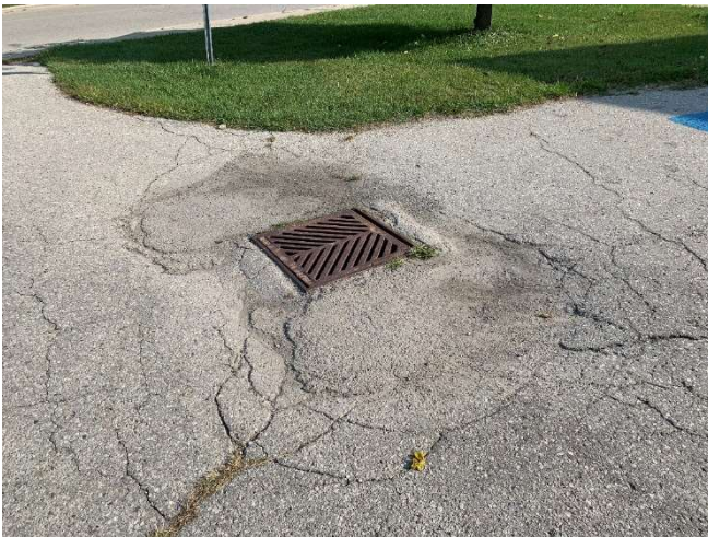
Settlement surrounding the catch basins was typical.
