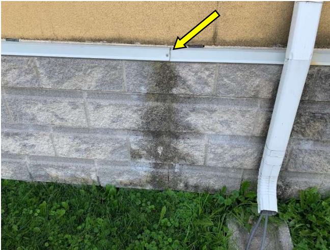
A leaky joint at the wall drip-edge is causing moisture staining/damage on the exterior masonry.
