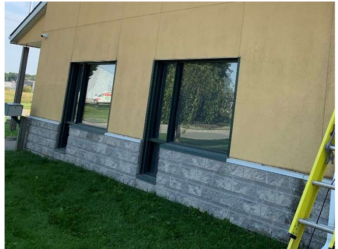
View of the typical aluminum framed windows with fixed configurations with double glazed panels.
