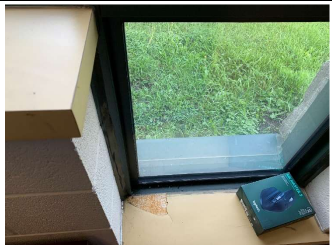
Water damage was observed at the windowsill in the fingerprint room.
