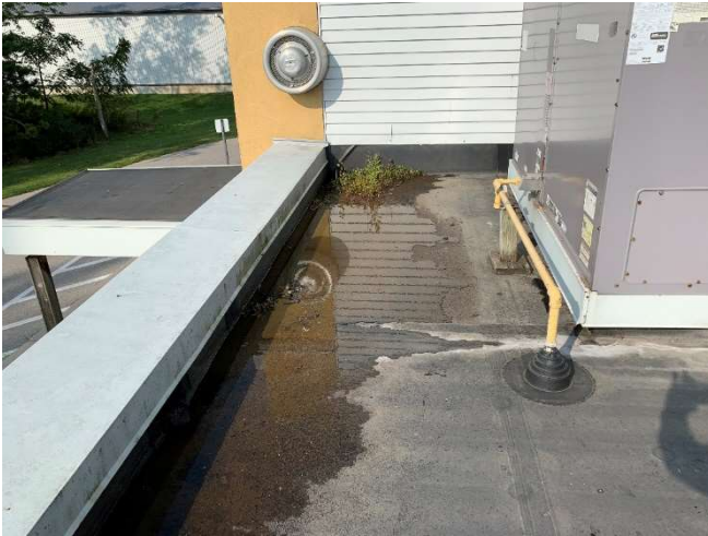
Water ponding and vegetation growth was observed at the south end of the building.
