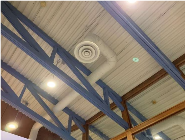
Exposed HVAC ductwork observed in the meeting room.
