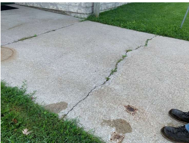
Cracking in the concrete walkways was noted at various locations around the site.
