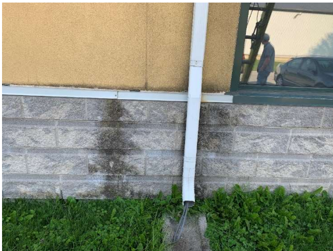
The split faced concrete block masonry was noted to be stained with moisture at a few locations.
