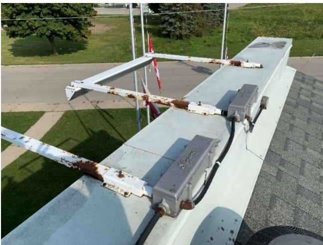
Corrosion was observed on the exterior light fixture brackets along the roof line at the west elevation entrance.
