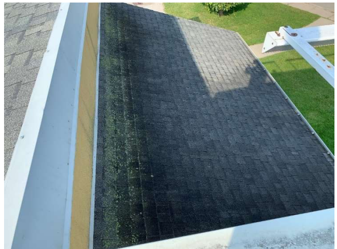
Saturated shingles with moss growth were observed on the asphalt shingles on the main entrance roof overhang.
