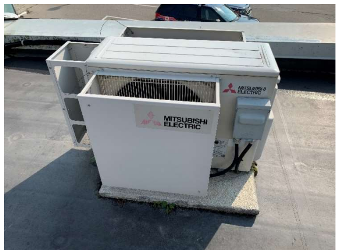
View of the split-system heat pump located on the low sloped roofing above the server room.
