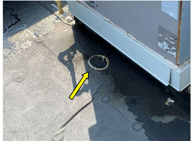
Patch repairs have been completed in previous years at the location of the ongoing leak above the cell block area.
