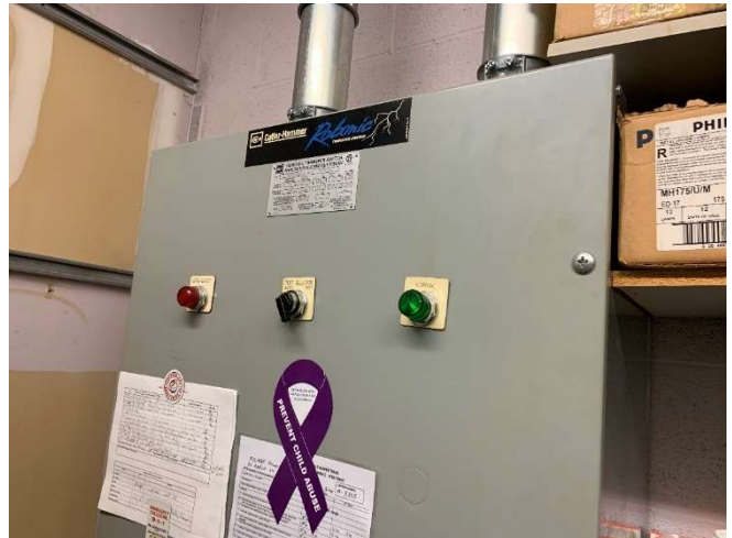
View of the automatic transfer switch located in the electrical room.
