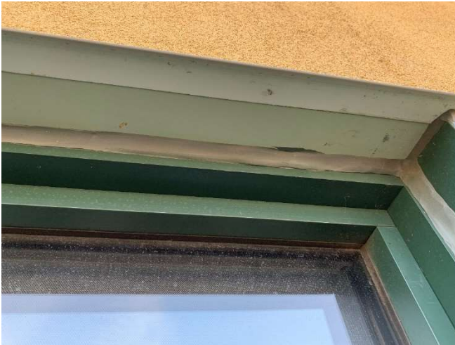
Close-up view of the perimeter sealant observed at a window head located along the west elevation.
