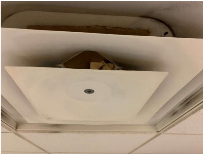
IRC observed that newspaper has been placed in the duct openings in some of the offices.
