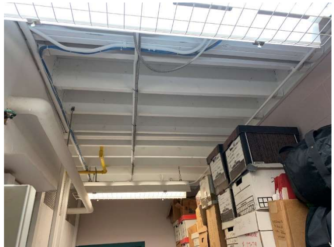
View of the wood roof joists below the wood decking observed in the evidence room.
