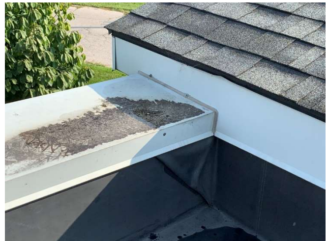
Moisture staining/debris accumulation were observed at the roof parapet flashings.
