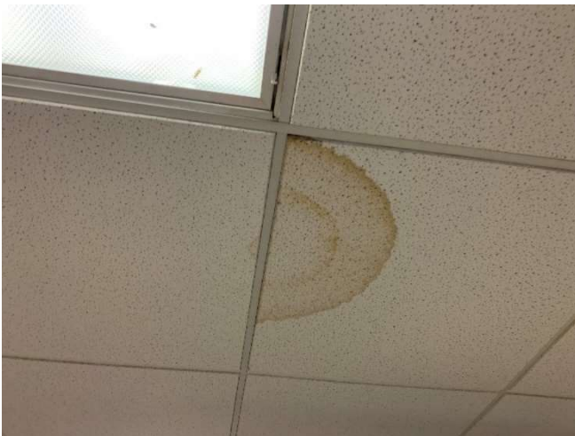
Stained ceiling tile observed in the fingerprint room.
