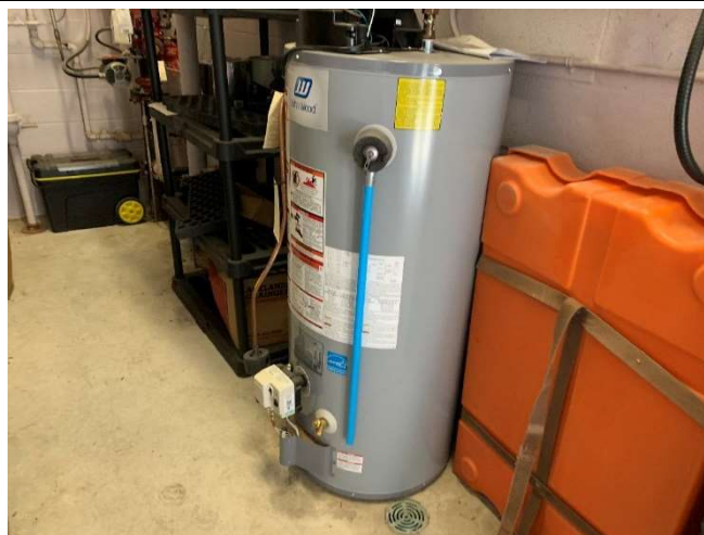
View of the automatic storage water heater.
