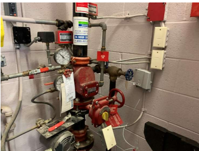
View of the sprinkler standpipe and valve system.
