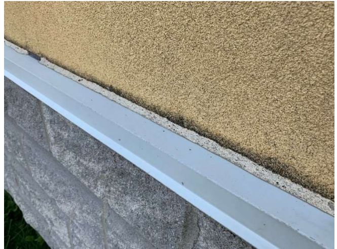
The caulking at the EIFS transition to the split faced concrete block was observed to be in poor condition.
