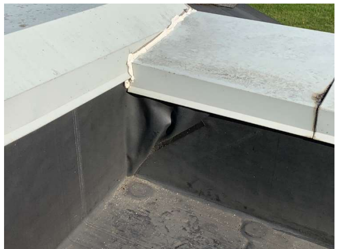
Evidence of poor installation in the form of wrinkling was observed in the EPDM roofing system.
