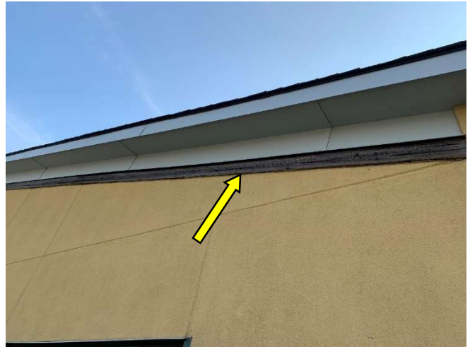
The wood trim has surpassed the serviceable life and replacement with metal flashing is recommended.
