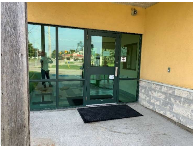
View of the hollow metal window wall system located at the main entrance vestibule.
