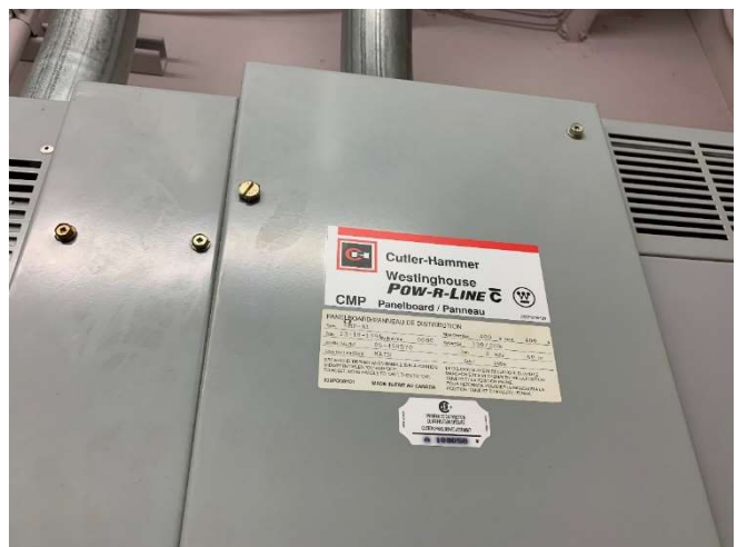
Close-up view of the main breaker panel manufactured by Cutler-Hammer.
