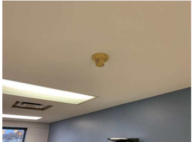
Heat sensors were observed at some locations but have surpassed the recommended serviceable life.
