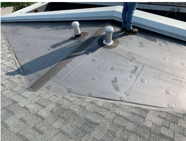
View of the single-ply EPDM membrane system observed on the low slope portions of the roof.
