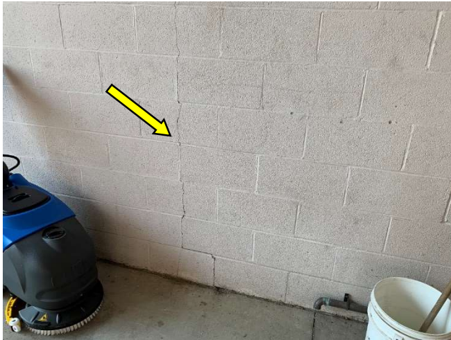
Cracking was observed at an exposed section of concrete masonry unit walls in the attached garage.
