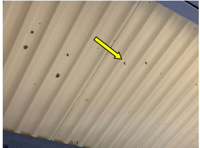
IRC observed shingle roofing nails through the exposed sections of the underside of the metal roof decking.
