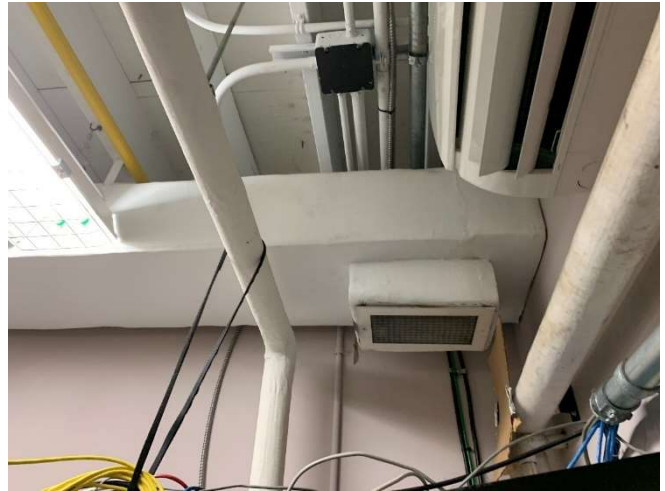
The HVAC ductwork was observed to be insulated.
