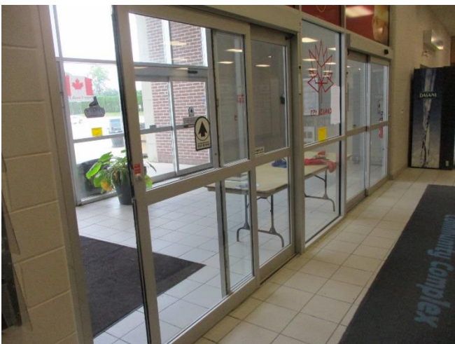
Flooring at the main entrance was in fair condition.
