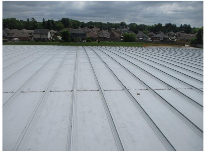
General view of the standing seam metal roof (Roof A).
