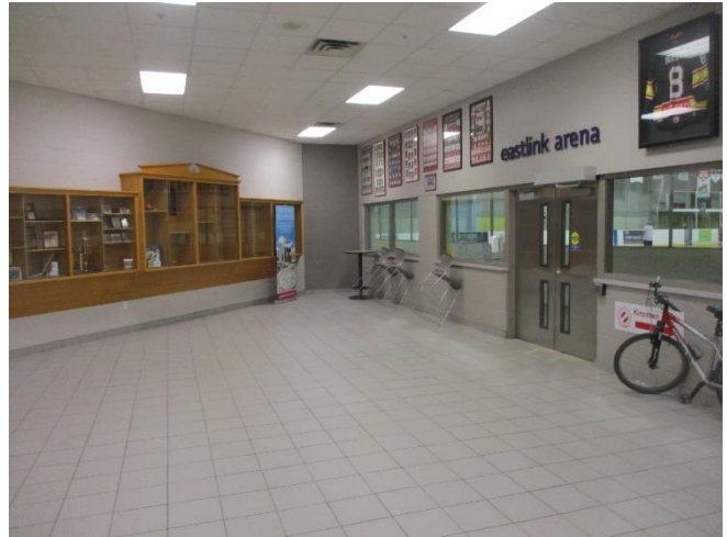
Interior drywall and doors at the main floor.
