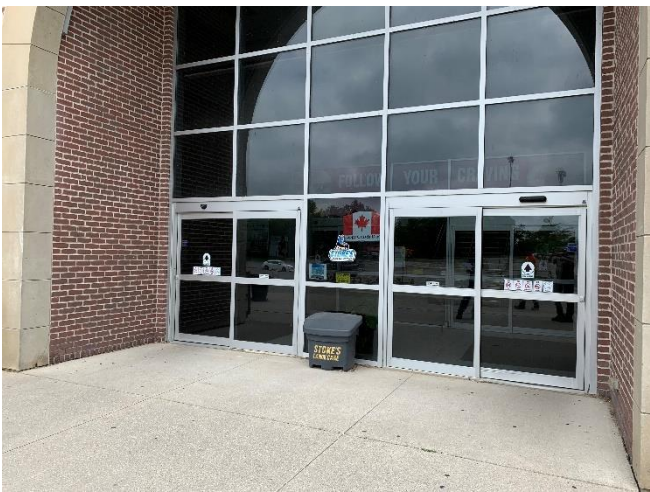
Exterior view of the main entrance glazing.
