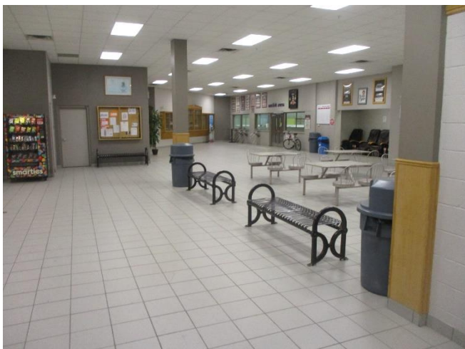
Floors, walls and ceiling finishes at the main level.
