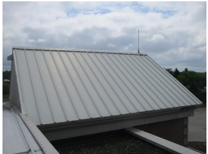
Roof B: General view of the prefinished metal roof.
