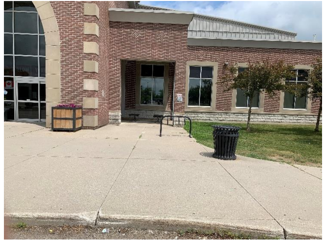
Pedestrian paving was noted in fair condition.
