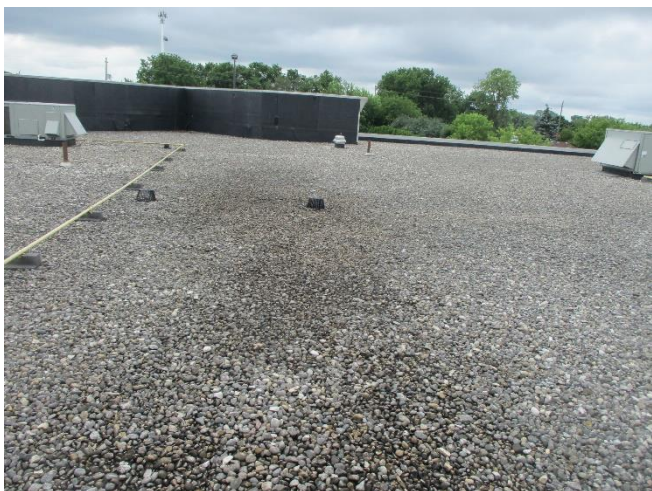
Roof C1.1: General view of the ballasted EPDM roof.
