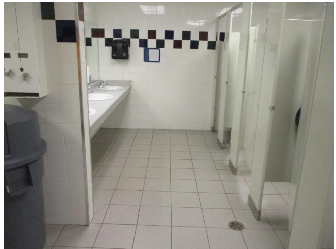
Finishes within a typical public washroom.
