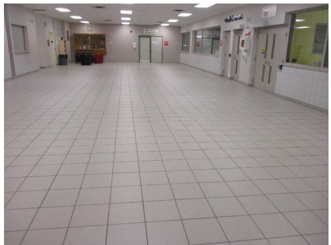
Flooring at the main level.
