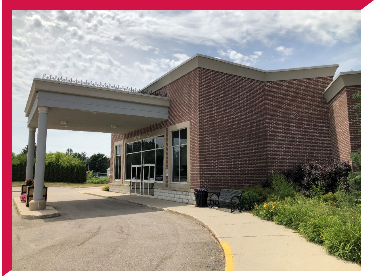
Figure 25: East Elgin Community Complex
