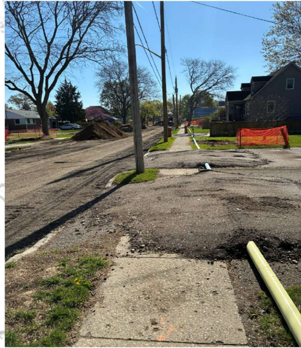
South Street – Temporary Waterline Installation
