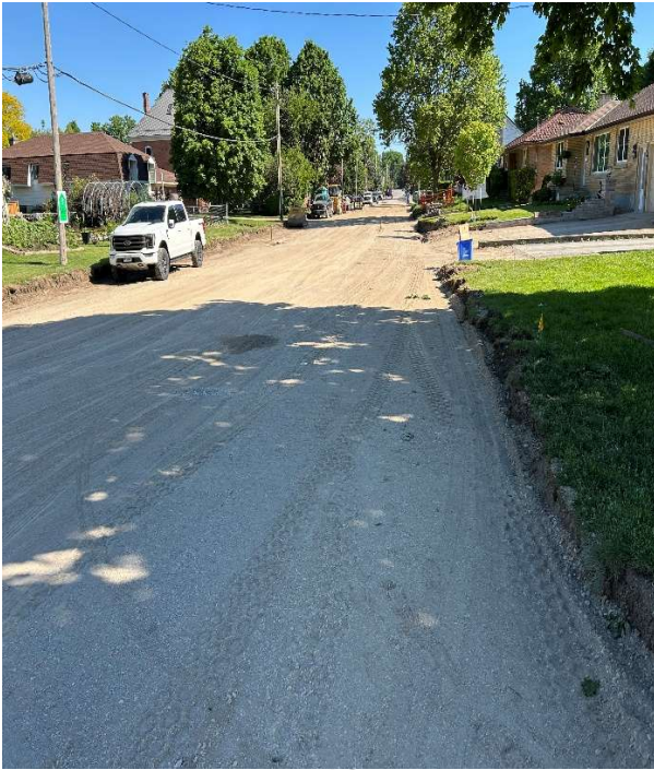
Victoria Street - Removals and Backfilled
