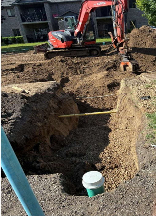
South Street – Installation of Sanitary Services
