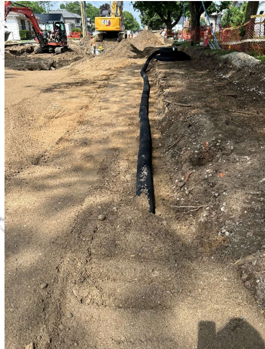
South Street – Drainage Tile
